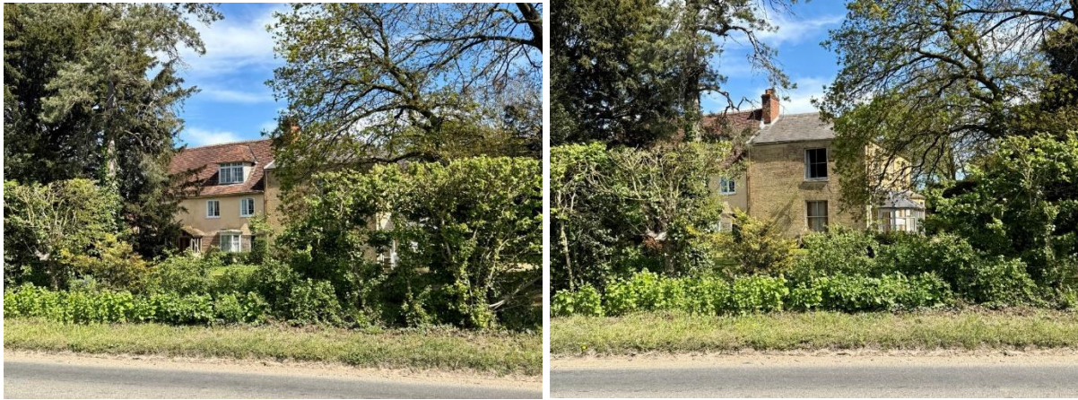
162 & 163: Views of the Old Rectory seen through surrounding mature trees looking east from Norwich Road
