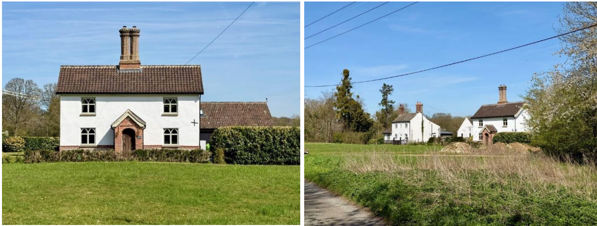
127 & 128: Setting to north and north-west with Holly Cottage set back from The Green
