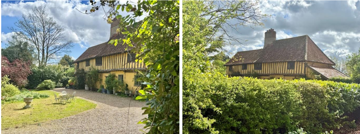
52 & 53: View of the Old Rectory looking east from within the churchyard
