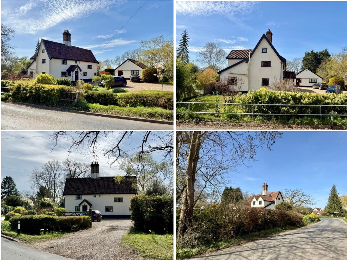
110-113: Setting of Manor Cottage in views to the south, west and north from the road
