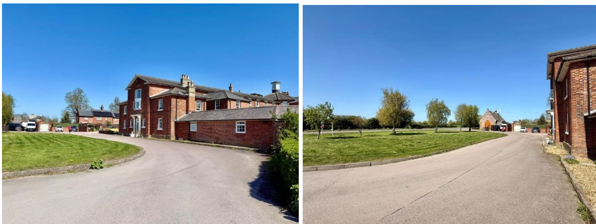
28 & 29: West façade of Hill House and open setting to the north and west
